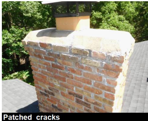
Patched cracks
