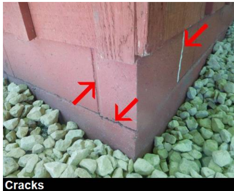
Crack with displacement
