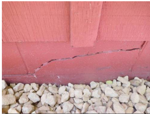
Crack with displacement
