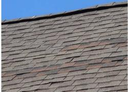
**Description:** Estimated total of 455 squares of laminated asphalt shingles over a membrane.
