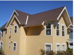
**Description:** Estimated total of 56,250 square feet of cementitious lap siding and hard board products installed as fascia, soffit, paneling, and window and door trim.
