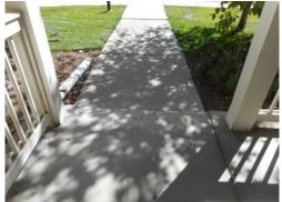
**Description:** Estimated 2,900 square feet of concrete approaches, presumed to be 6 inches thick and reinforced.
