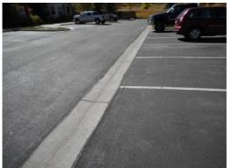
**Description:** Estimated 800 linear feet of 2-foot wide, reinforced concrete pan, sloped to convey stormwater runoff.
