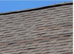
**Description:** Estimated total of 455 squares of laminated asphalt shingles over a membrane.
