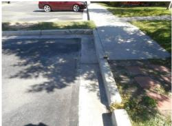
**Description:** Estimated 1,334 linear feet of 6 inch tall, spill and catch barrier concrete curbs with 1- and 2-foot wide gutters.
