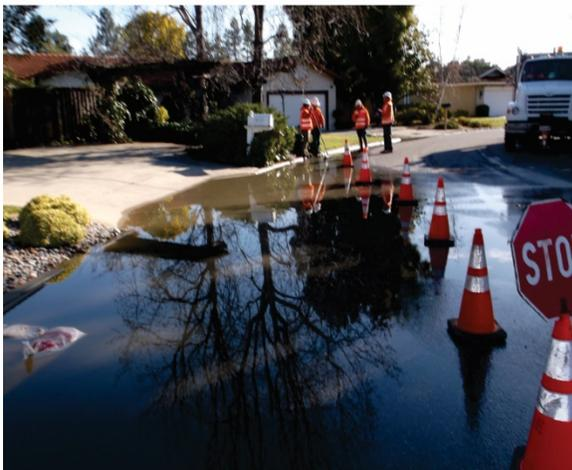
Sanitary sewer spills due to pump failure
