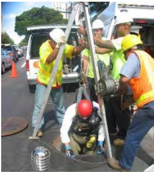
Photo 2-1. Confined Space Entry
