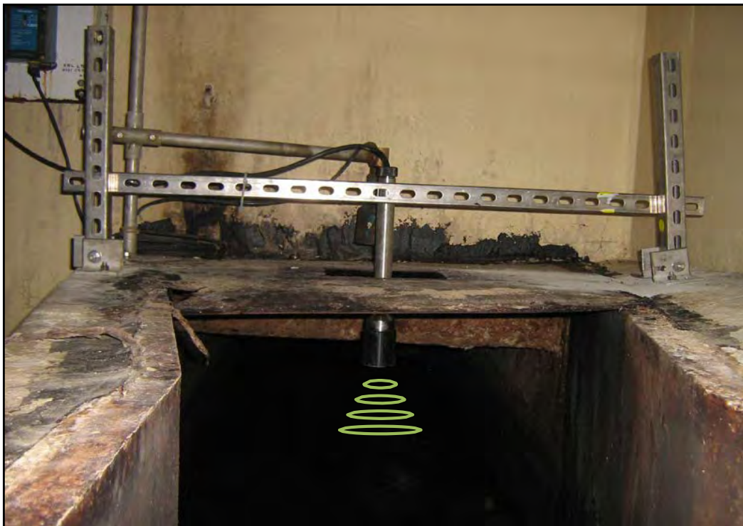
Figure 5. Parshall Flume Sensor Installation
