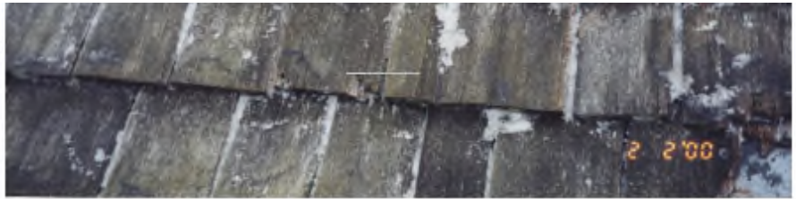
Original shingles installed on the roof systems north slope.
