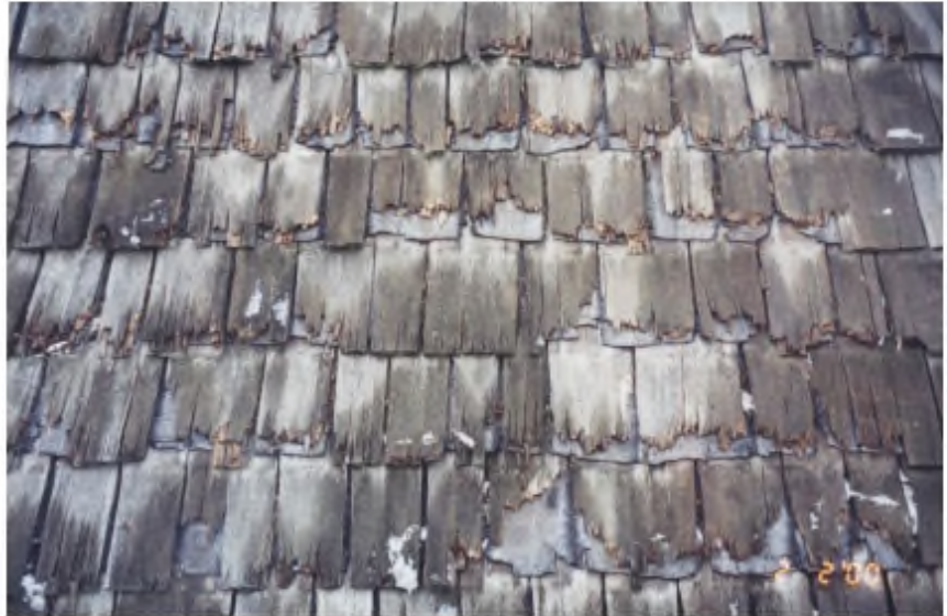
Original shingles installed on the roof systems north slope.
